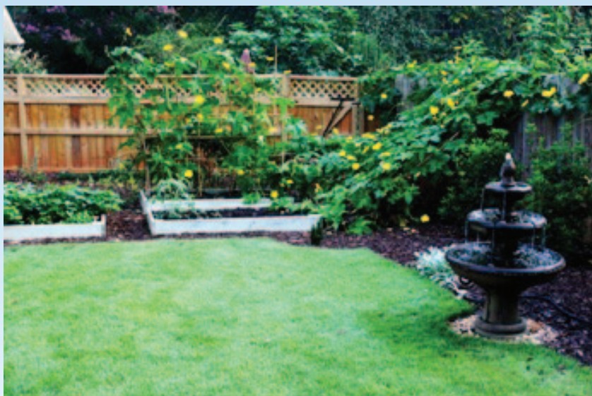
The ECOVIE rainwater collection system is located underneath the lawn.
