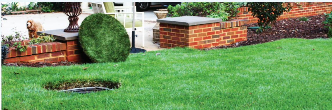
Access point to the underground collection unit
