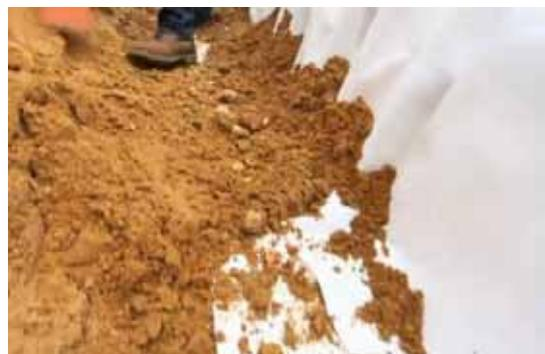
Image 11: Backfilling filter fabric for fixing
