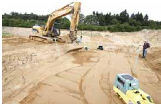
Image 13: Covering the tunnel elements
