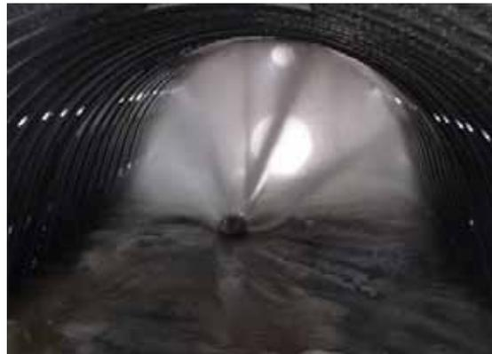
Image 4: Flushing nozzle with cleaning procedure
