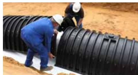
Image 9: Form lock fixing of two tunnel elements by overlapping
