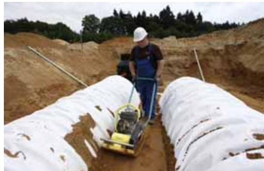
Image 12: Compacting with a small compacting device between rows of tunnel
