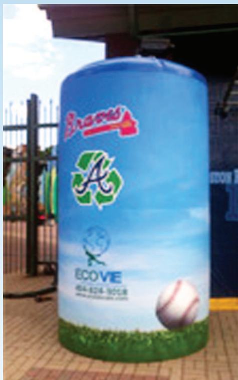
Installed System within Plaza area.
