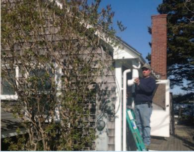
Ecovie designed a potable rainwater system to meet all water needs during the summer months. We provided all drawings, instructions, equipment, and phone/email support for our client to have the system installed using local trades people. The 2,000 gallon system has sediment and carbon filtration and UV treatment to assure excellent water quality with a design that has minimal maintenance requirements. The system is up and running with no more brackish water to deal with.
