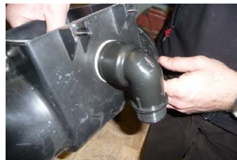
Fig. 4: Installed 90° connection bend
